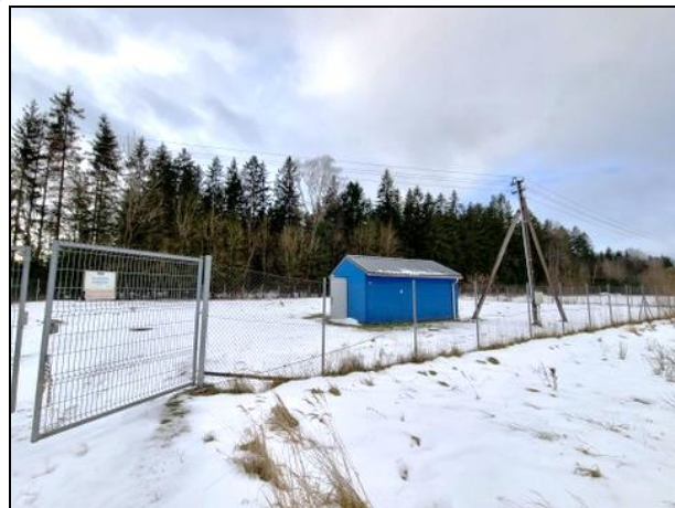
Vandens gerinimo stoties fasado fragmentai
